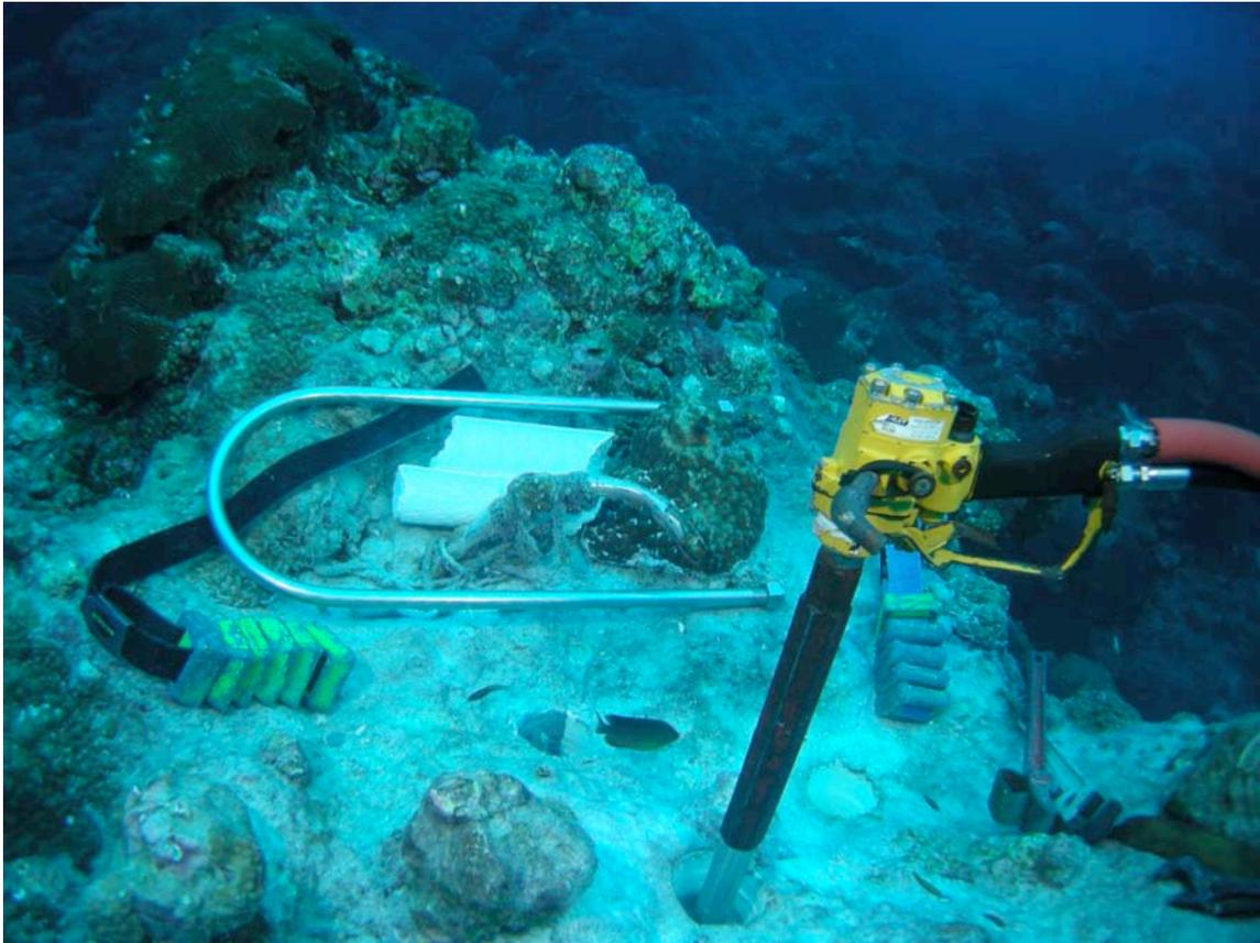
*Hydraulic drill rig sitting in one of a pair of holes drilled into dead coral at West Flower Garden Bank for Buoy #3. The new U-bolt sits in the background next to the old U-bolt, which has been twisted and broken. Coral cores which have been removed during the drilling process are also visible. The weight belts are used by the drillers to provide extra downward weight during the drilling process.*
